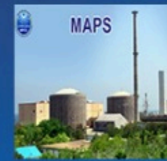
Madras Atomic Power Station, Kalpakkam 5 Camps in Kanchipuram, Tamil Nadu 4 Camps in Chengalpattu, Tamil Nadu
